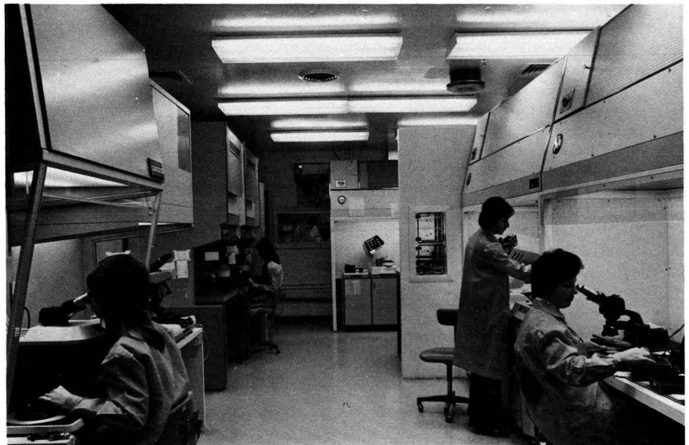
*Mask alignment is the key to the integrated circuit photolithographic process. The alignment machines shown here align IC circuit patterns to within 0.0001 inch (one-tenth of one-thousandth of an inch).*
