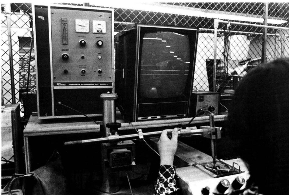
*Active abrasive trimming trims the resistor networks in our modular converters while the units are under power and operating. The precision of this trimmer, which we designed, allows high performance units to be built at a rate required for budget pricing.*
