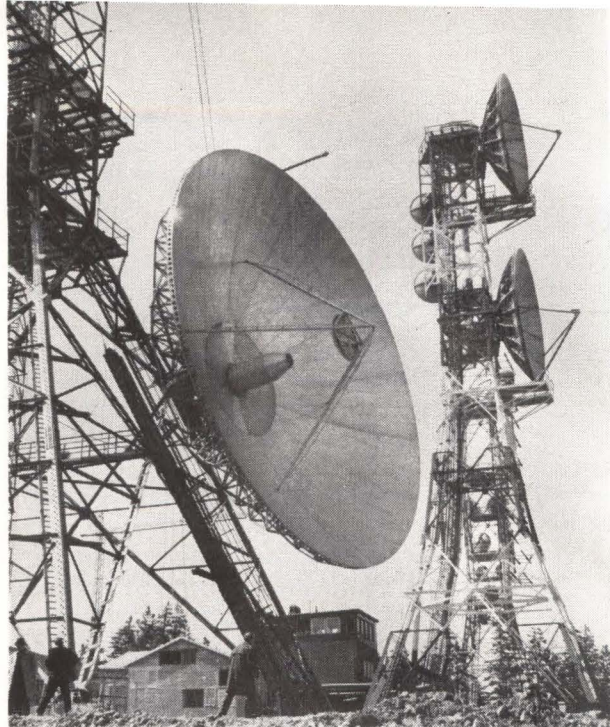
German Federal Post Office will have 100-mile Telefunken-built microwave link between West Germany and West Berlin in full operation by mid-1967. But cutback in Post Office budget for communications will depress microwave market next year.
