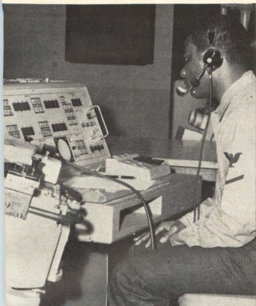
War games. With this console, operator can position six surface or subsurface targets within a given operations area.
