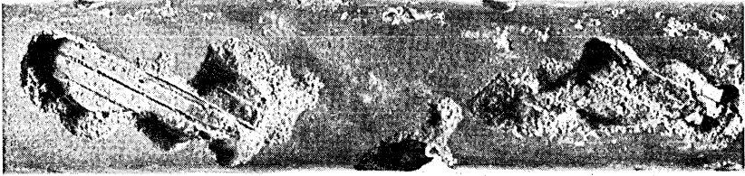
Fig. 5—Underground wire damaged by insects after two years of service in Decatur, Alabama.
