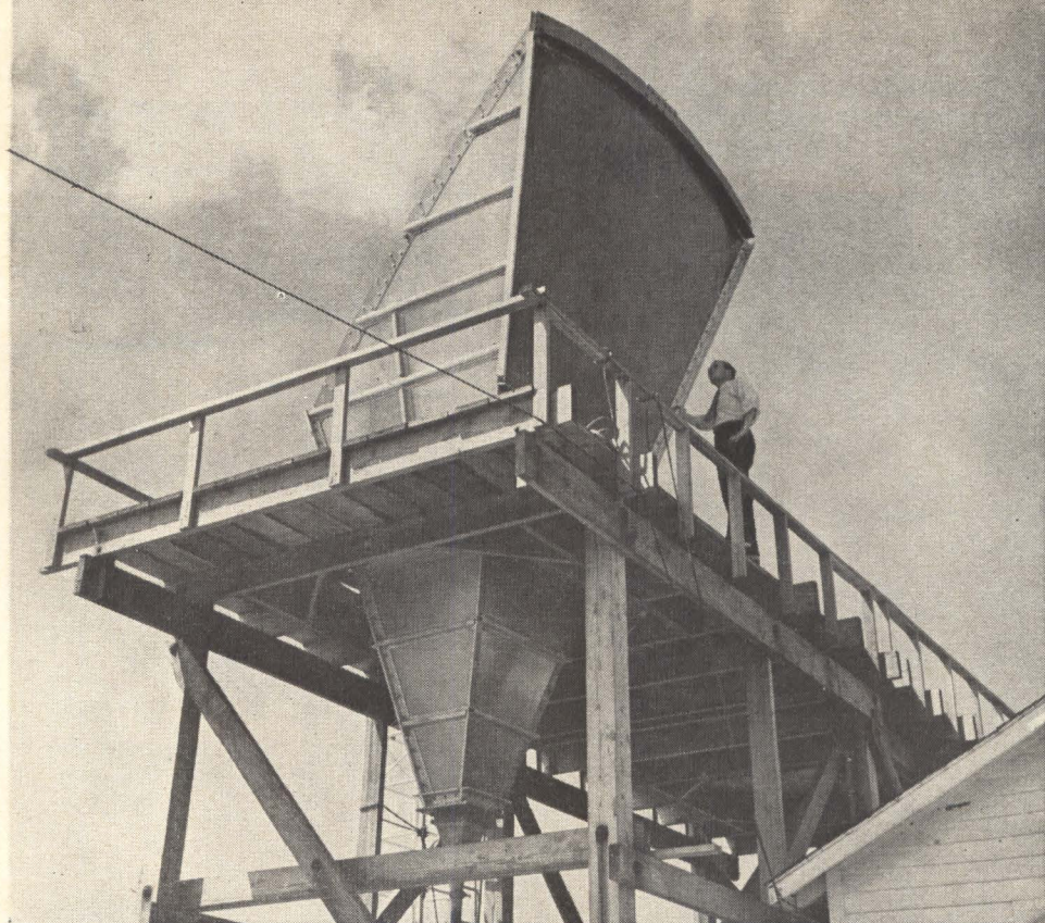
FIG. 3—Horn antenna handles signals in the 4, 6 and 11 Gc bands simultaneously
