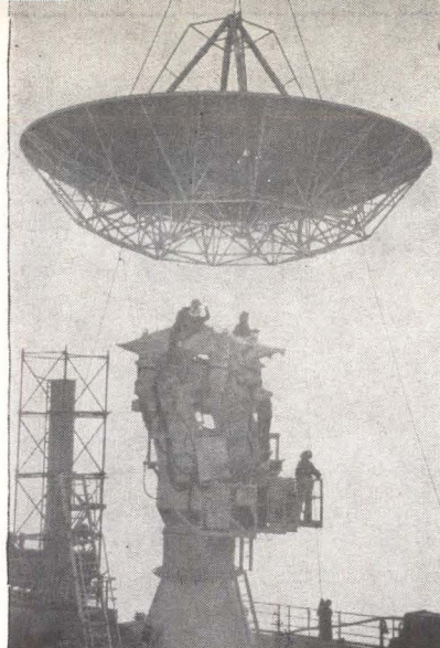
SYNCOM TESTS will be made by USNS Kingsport, off Nigeria, and station at Lakehurst, N.J. Photos show installation of 30-foot Triax antenna, by GE, and control room. Bendix headed team equipping the ship
