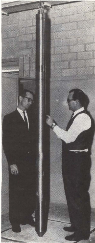
SEISMOMETER for use in holes or wells as deep as 10,000 ft improves signal-to-noise ratio as much as 10:1 over surface types
