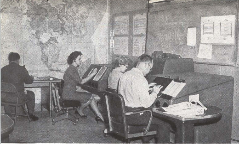
HIGH RESOLUTION, motorized film viewers for seismic analysis program compare two seismic signals. Digital and analog computers are also used in analysis
