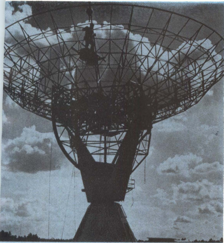
TRACKING ANTENNA designed for Air Force by Radiation, Inc., with receiving bandwidth of 100-2,300 Mc, is part of a $1.5-million contract. Antenna systems will be installed at both the Atlantic and Pacific missile ranges
