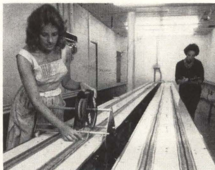
DIODE BURN-IN to improve semiconductor reliability at Sperry Rand Corp. Units are subjected to many hours of electrical stress. Diodes will be used in Polaris missile
