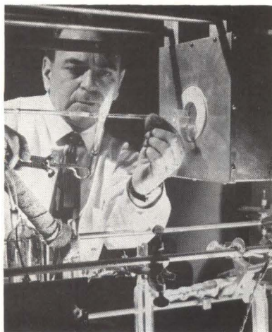
ABSORPTION CELL containing mercury isotope is sealed
