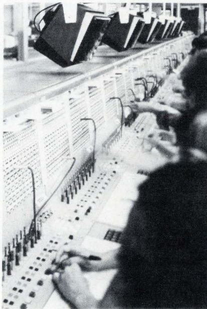
Call manager. TI's long-distance control system uses minicomputer to schedule calls.
