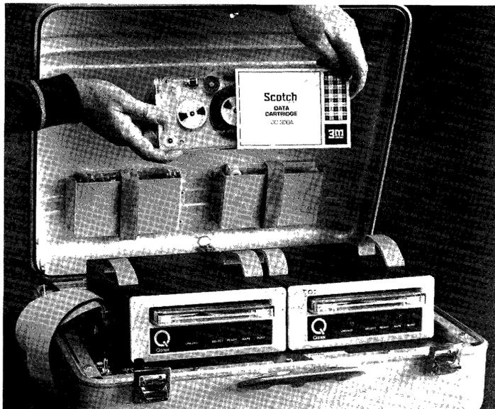
North Atlantic's Qantex Division announces the dual Model 2710 portable digital cartridge recorder, featuring a complete and autonomous data storage system that uses the 3M DC300A Data Cartridge as the tape storage medium. The recorder comes with interfaces for DEC PDP-11, DEC LSI-11, Nova, and other popular minicomputers, as well as the Intel 8080 microprocessor, and includes power supplies, formatter, and interconnecting cables.
