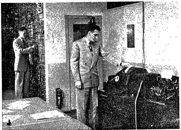
Figure 4. Operators making step-by-step check of teletype input-output facilities
