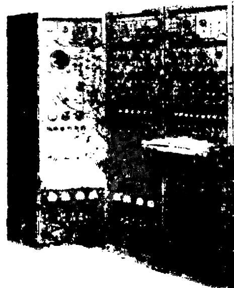
Figure 6-96. Typical analog-computer installation in which patching is accomplished by the use of cabling between components.
