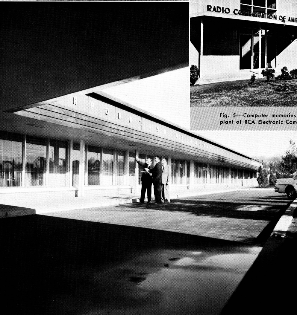
Fig. 6—Engineering and production of computer circuit devices and microcircuits is centered at this Somerville, N.J. plant of RCA Electronic Components and Devices.
