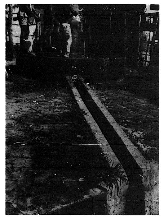
STANDPOST WASTE WATER DRAINAGE CHANNEL
