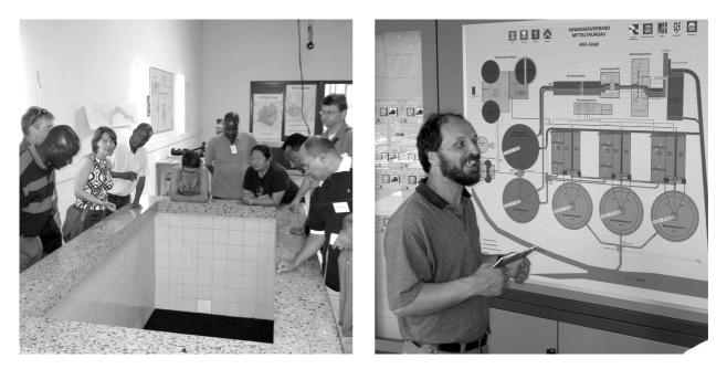
In the *control room* of the Technische Betriebe Weinfelden all relevant information for the water supply, natural gas, electricity and communication is collected electronically and can be accessed via computer stations. In case of a problem the system automatically raises an alarm and informs the staff member on duty. This staff member has afterwards to confirm the alarm and is subsequently fully responsible to settle the emergency.
