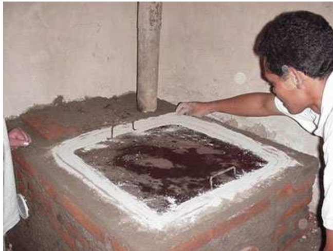
Justa Stove: sealing the plancha
