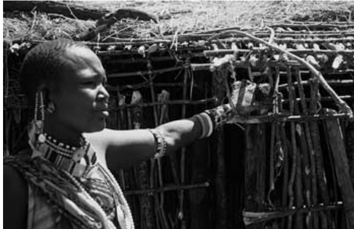
A builder pauses by the structural framework of her traditional house before plastering it. Photo: Practical Action / Lucky Lowe.
