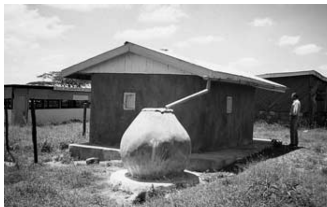
At the Maasai Rural Training Centre demonstration site, Practical Action staff and local artisans, built four new types of housing enabling skills to be developed and providing physical evidence for others to see. Photo: Practical Action / Dave Mather.
