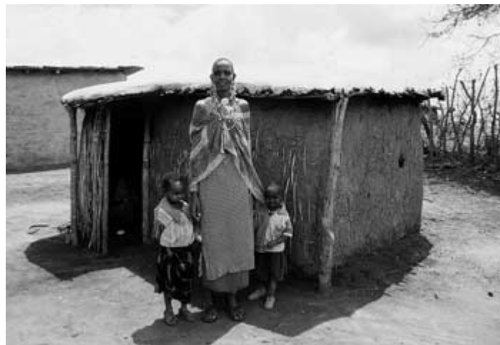
Mrs Silole Malipe Empariya built her own ferro-cement skin roof. Photo: Practical Action / Lucky Lowe.
