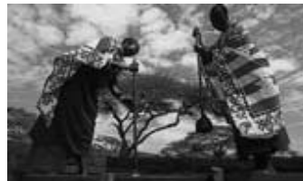
Maasai women being trained whilst preparing and moulding rammed earth walling. Photos: Practical Action / Neil Cooper.
