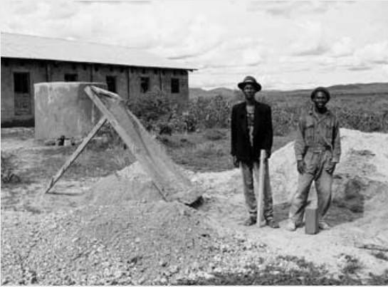
Amos Sikishoi and his assistant Olongida Molel in front of the new girls' dormitory being built at Ibisil Primary School. Photo: Practical Action.
