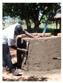
The DRIP tank is a fired brick built cylindrical tank standing on a base of approximately 1.5m diameter.
