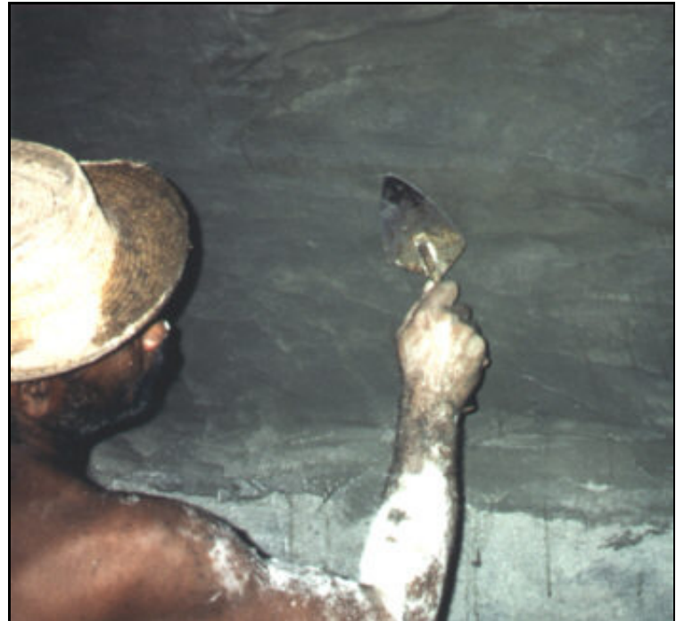
Inside plaster of the gastight section of a fixed dome digester
