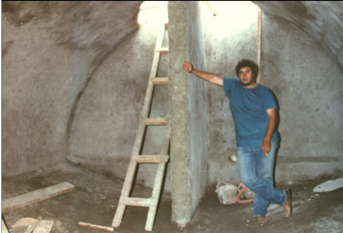
View in a canal digester, Burundi
