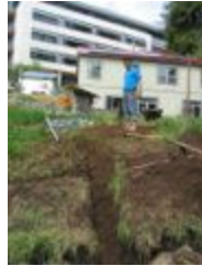
Fig 12f: Covering piping with soil
