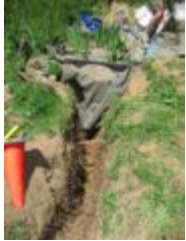
Fig 7e: Irrigation trenching begins
