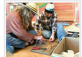
Thorin and Bart Working on some wiring
