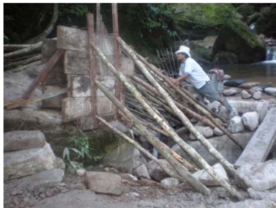
Figure 3: Civil engineering for a micro hydro scheme in Bocatoma, Peru. Photo: Soluciones Prácticas.
