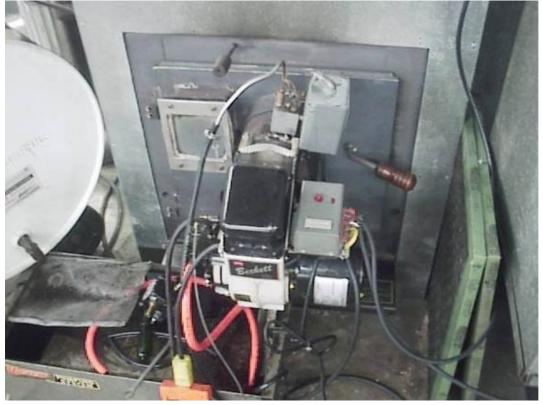
the eye input and a set of contacts for the thermostat. In the plenum I have a temp probe from a water heater that interrupts the burn cycle if the air temp goes over 200 F. Notice the pre-heater block for the oil with a waterheater-
