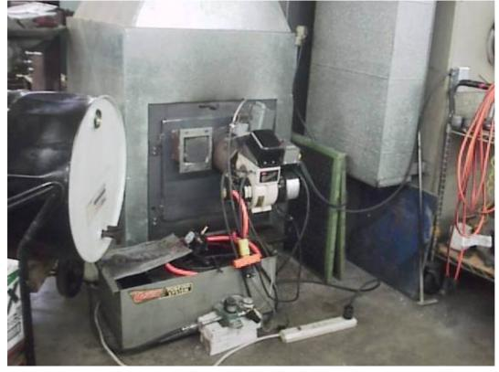
System on 01/09/03 Shows Duct shroud around woodstove with new door outfitted with the retro-bab and a window to view the flame.
