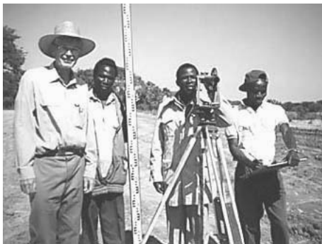
Fr. Otten and crew survey the site for an earthen dam that stabilized the water supply for wheat farmers in Zambia.
