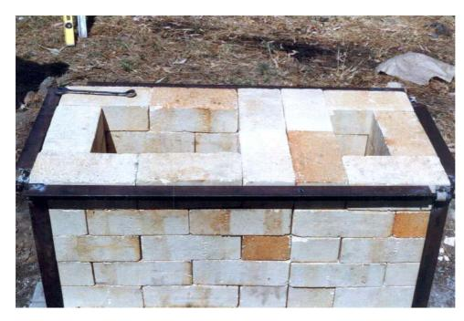
Figure 4: Tie-bar arrangement
