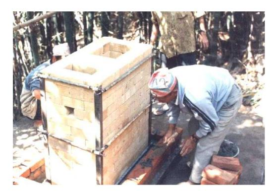
Figure 5: Alternative tie-bar arrangement
