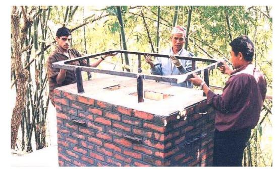
Figure 9: Fitting the top framework
