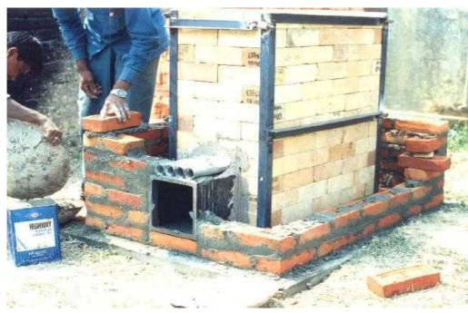
Figure 6: Air inlet pipes and ash door
