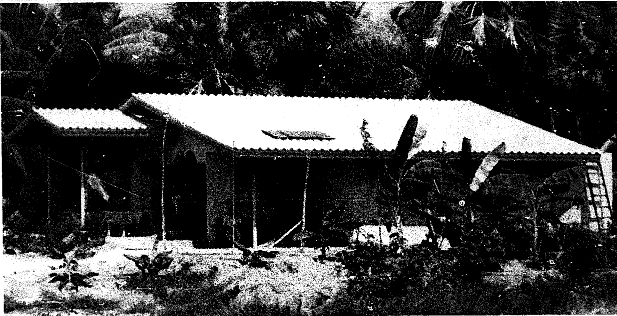
Figure 7.8 Lighting in a Rural Health Clinic
