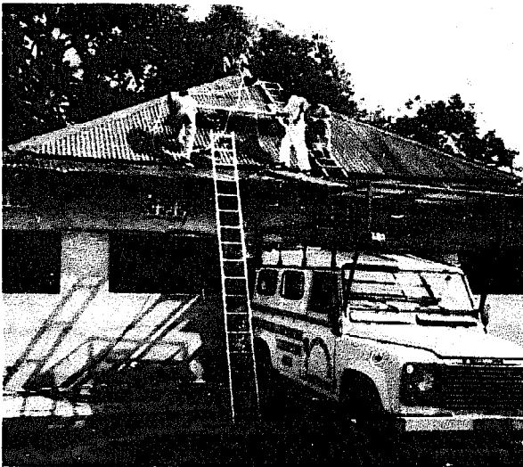
Figure 3.9 Carrying a PV Array onto a Roof
