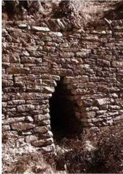
A dry masonry retaining wall with a scupper culvert
