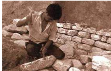
Dressing stone during the construction of dry stone dentition
