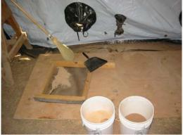
mosquito netting. The clay is dumped onto the sieve and then it is shaken onto a clean floor. The sifted material is then swept up with broom and dustpan and placed into a container for mixing.
