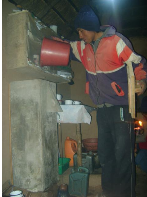
Figure 1: A domestic bio sand water filter being used in Peru. Photo: Soluciones Prácticas.
