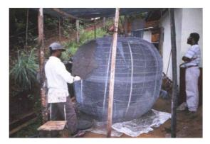
Figure 2: a) One of the 10 legs used to form the skeleton frame. b) The skeleton frame being rendered.
