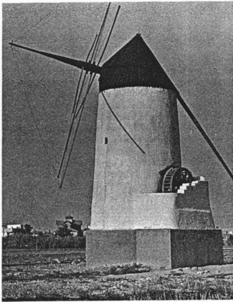
Left: High irrigation mill at El Algar. Top right: Sail spars at wind shaft. Bottom right: Noria, a well mechanism of Arab origin, at Mallorca. Long arm turned by blindfolded donkey or mule.
