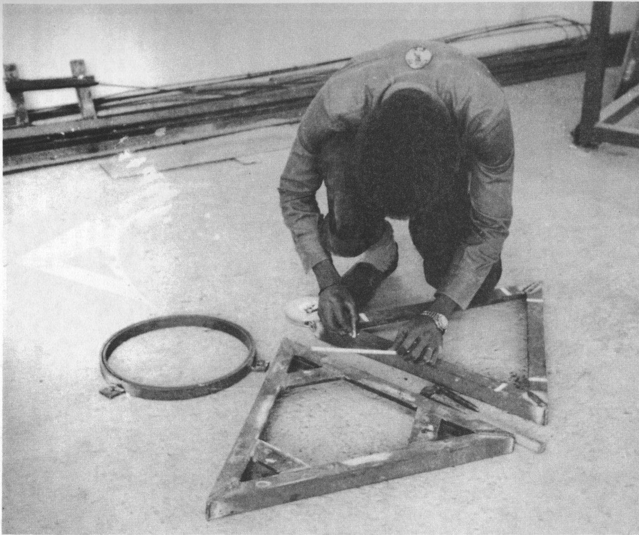
Making upper tower section frame.
