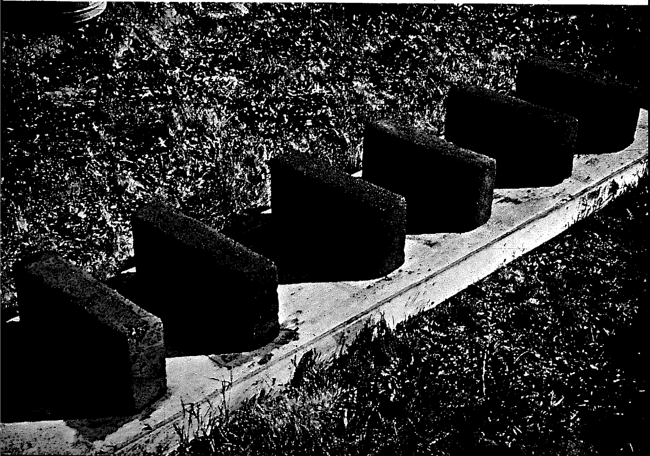
Drying bricks on edge.
