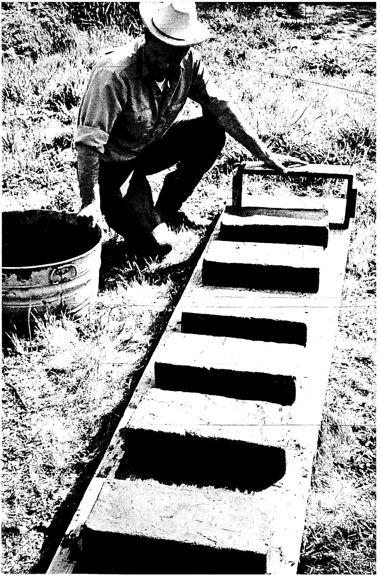
Drying bricks where they lay cast, for the first three or four days.
