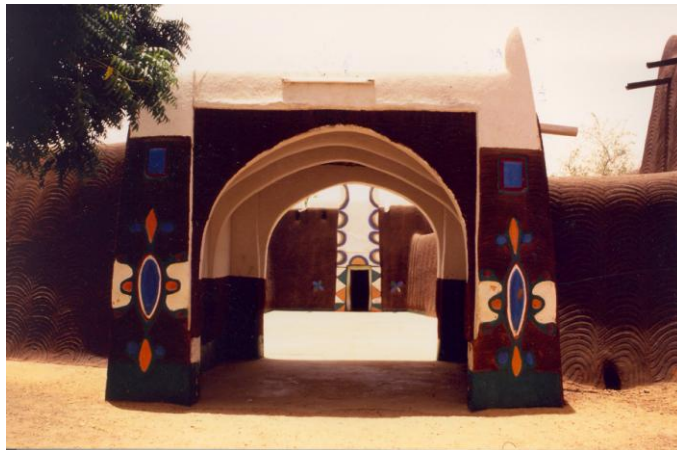
Figure 2: Soil-based render - stabilised with bark of Néré, Nigeria. Photo credit: CRATerre/EAG
