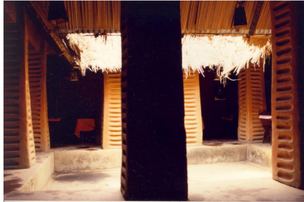
Figure 1 Surface stabilisation of soil with palm oil, Nigeria. Photo credit: CRATerre/EAG
