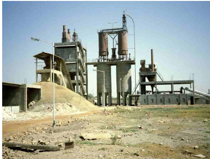
Figure 2: Medium-scale Portland cement plant, India Photo: Practical Action
