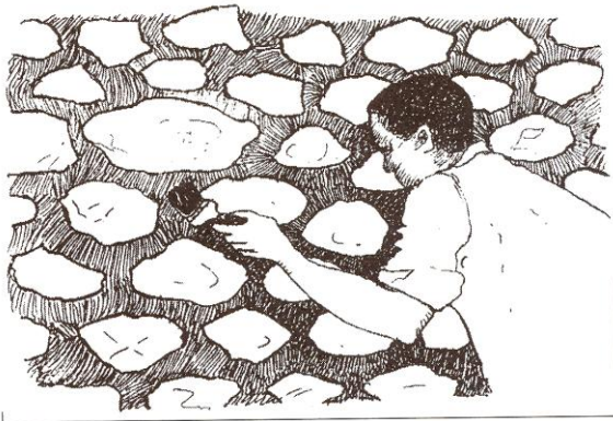
Figure 8: Brushing the joints with clean water must be done after each day's work.
