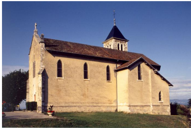
Figure 3: Church built in pisé (rammed earth) at Charancieu in the Dauphiné region of France. Photo: CRATerre/EAG
