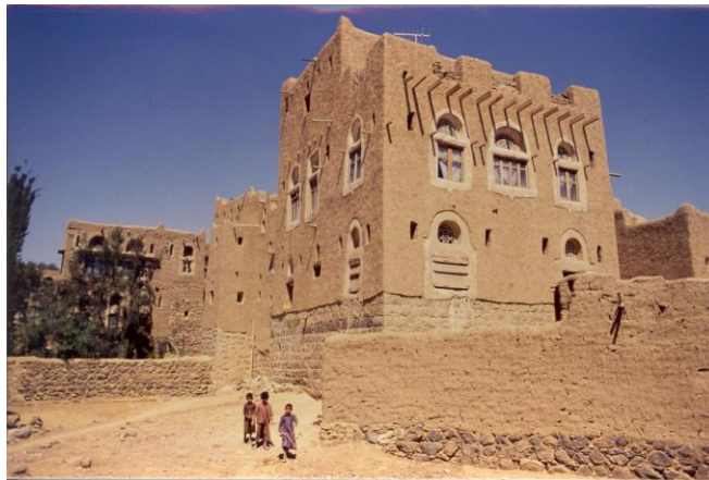
Figure 2: Private house built in the town of Amran in Yemen in 1985 Photo: CRATeere/EAG
