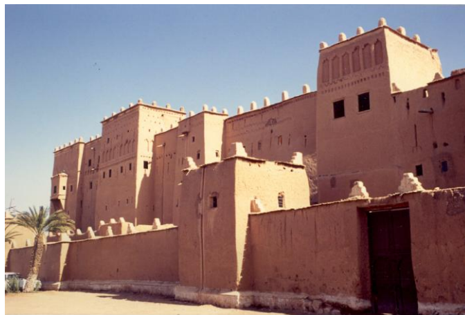
Figure 4: The Kasbah of the Glaoui at Ouarzazate in Morocco. Built by the beginning of the 20th century. Photo: CRATerre/EAG
