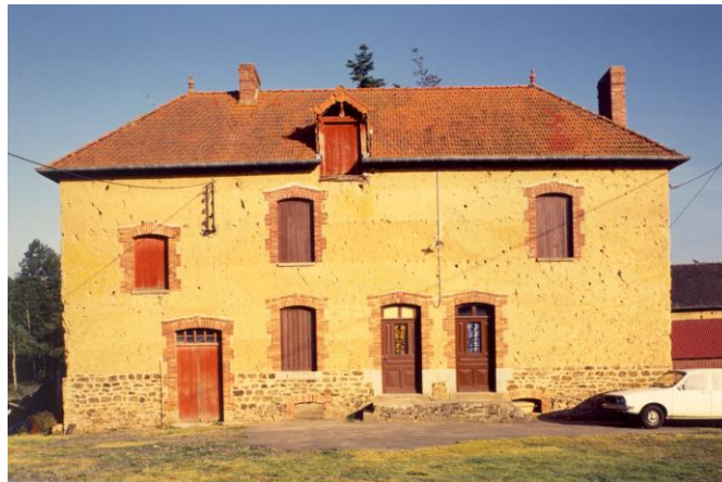
Figure 1: House near Rennes in France built at the end of the 19th Century Photo: CRATerre/EAG.
