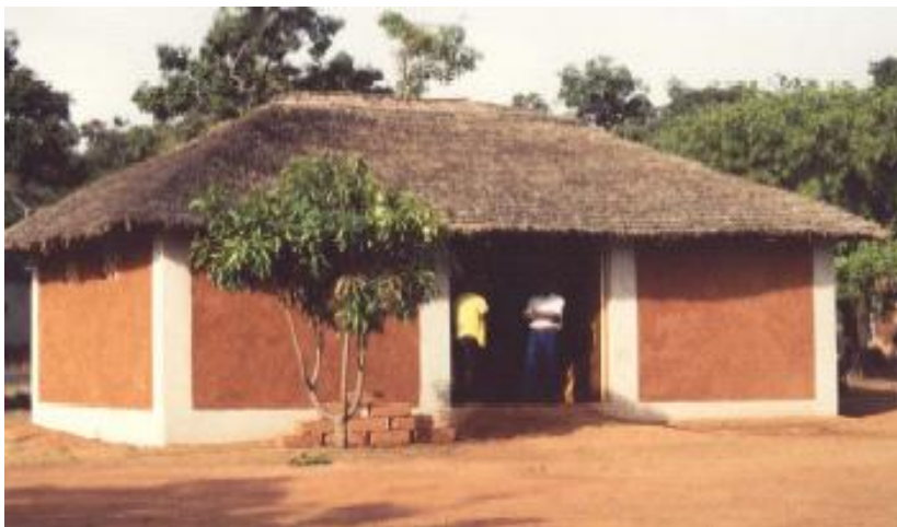
Figure 4: Demonstration house in Jos, Nigeria, built with adobe laid in mud mortar and plastered with mud mortar. Photo: CRATerre/EAG
