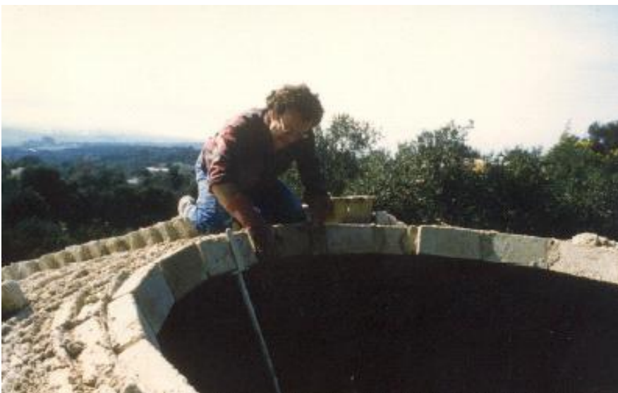
Figure 2: The good cohesion of mud mortar allows construction of vaults and cupolas without shuttering. Photo: CRATerra-EAG.
