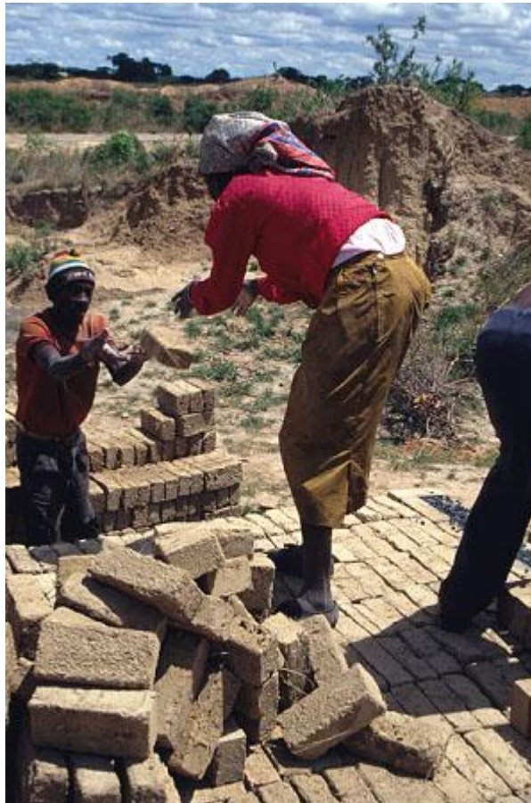
Figure 2: Brick makers are shown building the clamp kiln prior to firing, Zimbabwe. Photo: Practical Action / Janet Boston.
