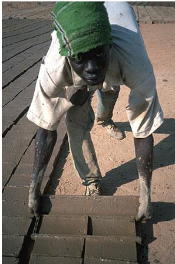
Figure 3: Brick-making using improved kiln at Kassala, Eastern Sudan. Releasing the moulds and laying bricks for drying. Photo: Practical Action / Mohammed Majzoub.
