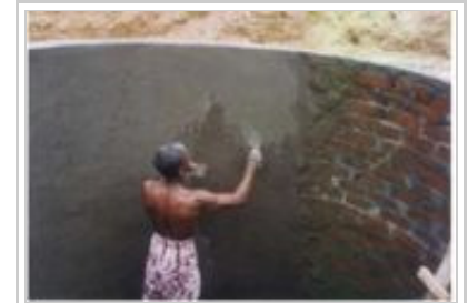
Fig 12: Plastering the tank
