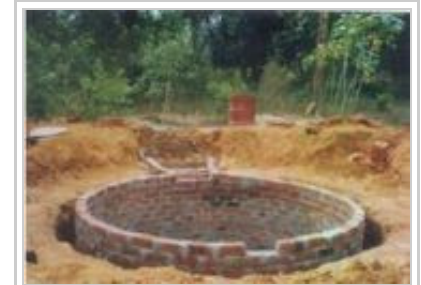
Fig 11: Completed tank before plastering
