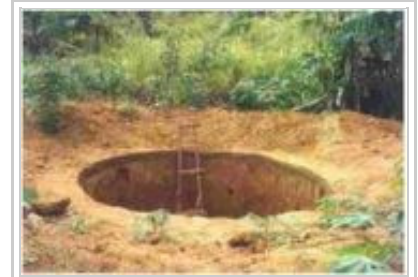
Fig 3: Pit for the tank construction
