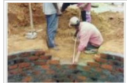
Fig 6: Measurement taken for the inlet construction.
