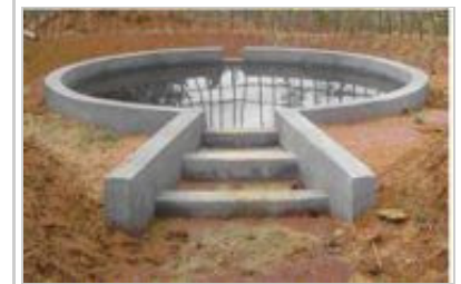
Fig 14: After the completion of the rainwater harvesting tank
