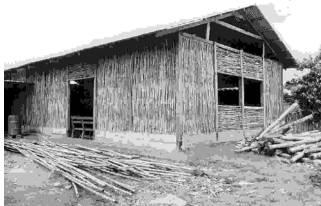
Figure 10: The Community building in Soritor during construction ©Practical Action /Rumi Velaccliaga
