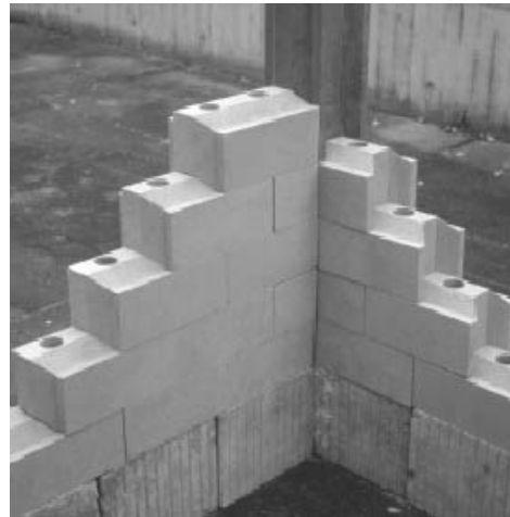
7-15 Improved interlocking system of FEB, Kassel, 2001
