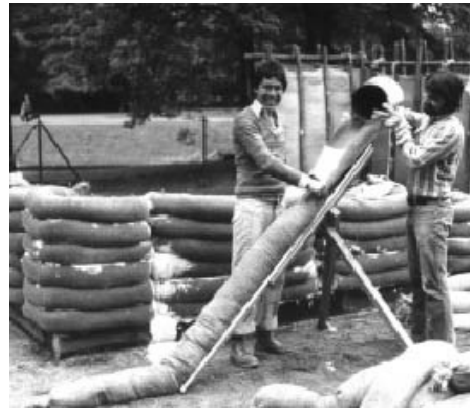
9-2 and 9-3 Wall with filled textile hoses
