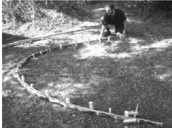
15-7 Construction of the arc with split bamboo
