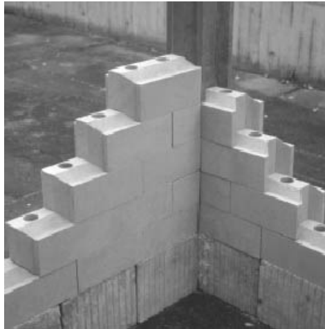
7-15 Improved interlocking system of FEB, Kassel, 2001
