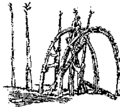
Mudhif (guest house) of the Ma'dan (Marsh Arabs), Iraq: bundled giant reeds as frame structure and scaffold, reed mats as cladding
