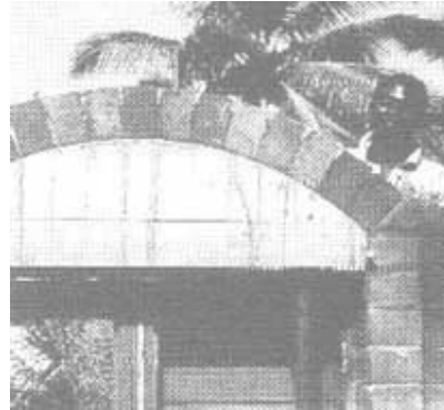
Wooden formwork
