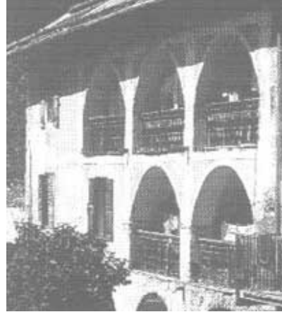
Farm building using several levels of ribbed vaults, Queyras, France
