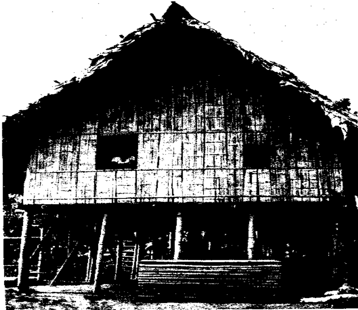
FIGURE 1--From supporting posts to rafters and sheathing, this cottage in the Ecuadoran lowlands is made entirely of native bamboo, Guadua angustifolia . The posts may serve for five years; the siding may remain in serviceable condition for decades.
