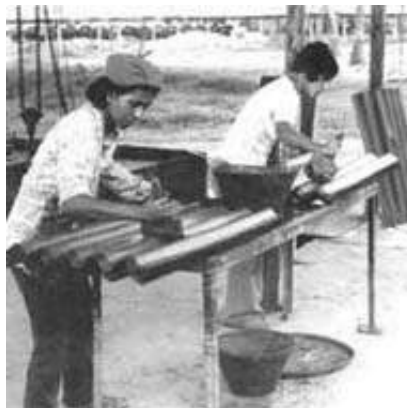
The final coat on asphalt roof sheets (Colombia)
