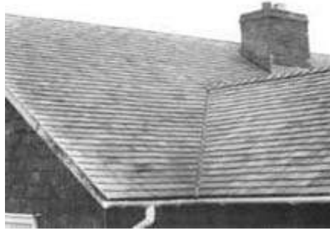
Shake roof and timber-clad walls
