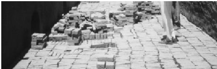
Fig 5: Stacking bricks for firing in a permanent brick clamp in Sudan.
