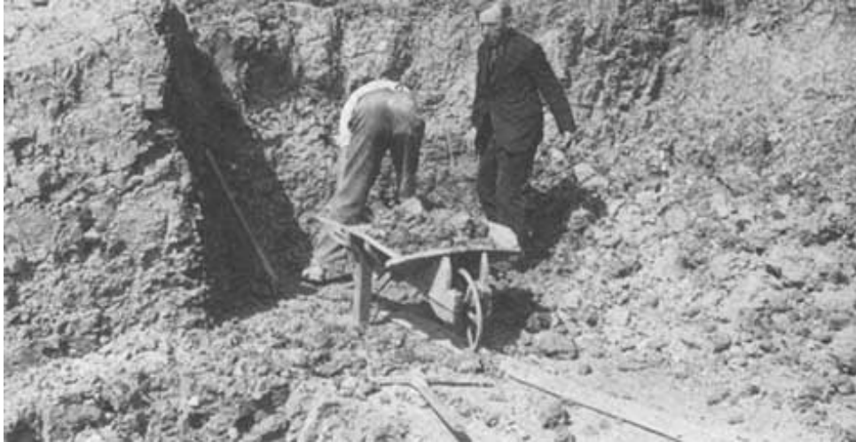
Figure III.3 - Digging and transporting of dry hard clay (United Kingdom)
