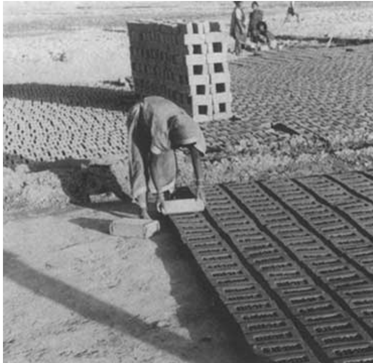
Figure V.11 - Two moulds demoulded at the drying ground. Good finish of produced bricks (India)
