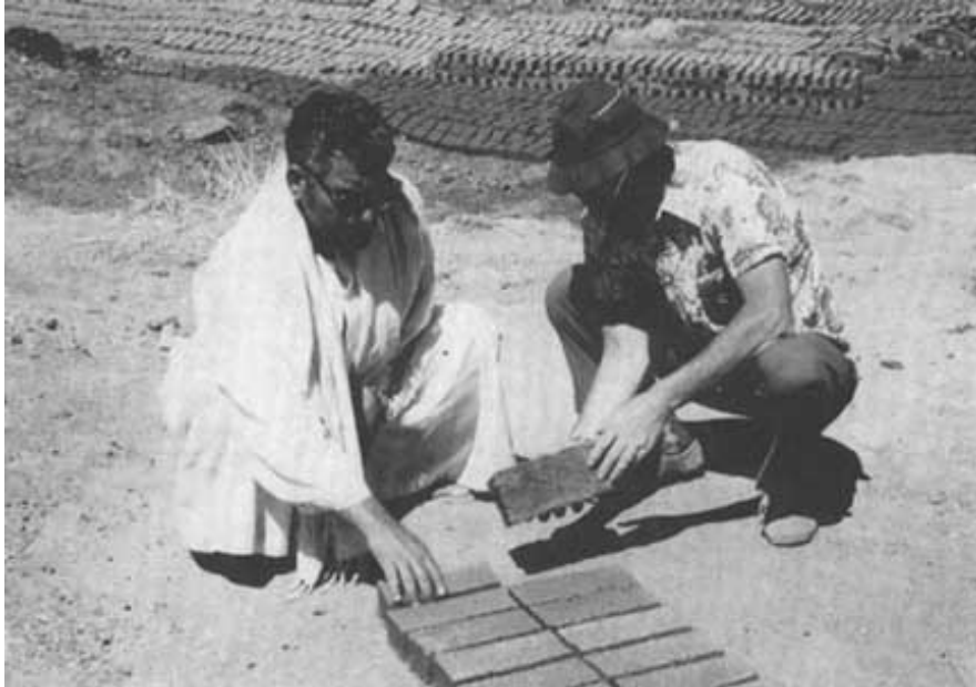
Figure VI.4 - Good bricks dried on clean, level ground (West Sudan)
