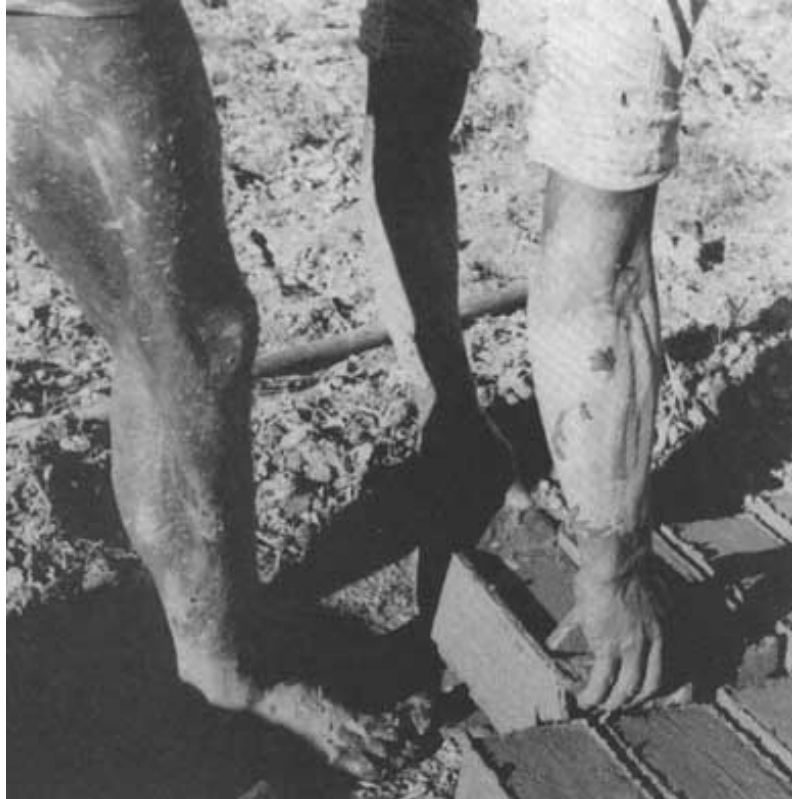
Figure V.9 - Demoulding by pushing on triangular end pieces (Madagascar)
